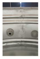
This is picture from the inside of the tank. Make sure the inlet with the raster is the lowest and the inlet with the hole is positioned the highest
