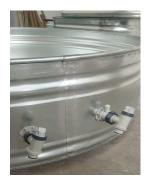
This is a picture from the outside of the tank. Both inlets with the valves connected, ready to connect the hoses with clamps.
